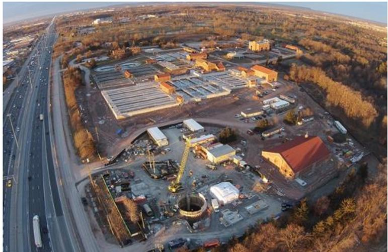
“Hatch is very honoured to be recognized with an Award of Excellence for the Mid Halton Wastewater Treatment Plant (WWTP), Micro-Hydro Facility project as it symbolizes sustainability, innovation and positive change. The micro-hydro system provides a source of sustainable power generation while reducing the carbon footprint and energy costs of the WWTP,” remarked Carl Bodimeade, P.Eng. Hatch’s Senior Vice President, Infrastructure.
