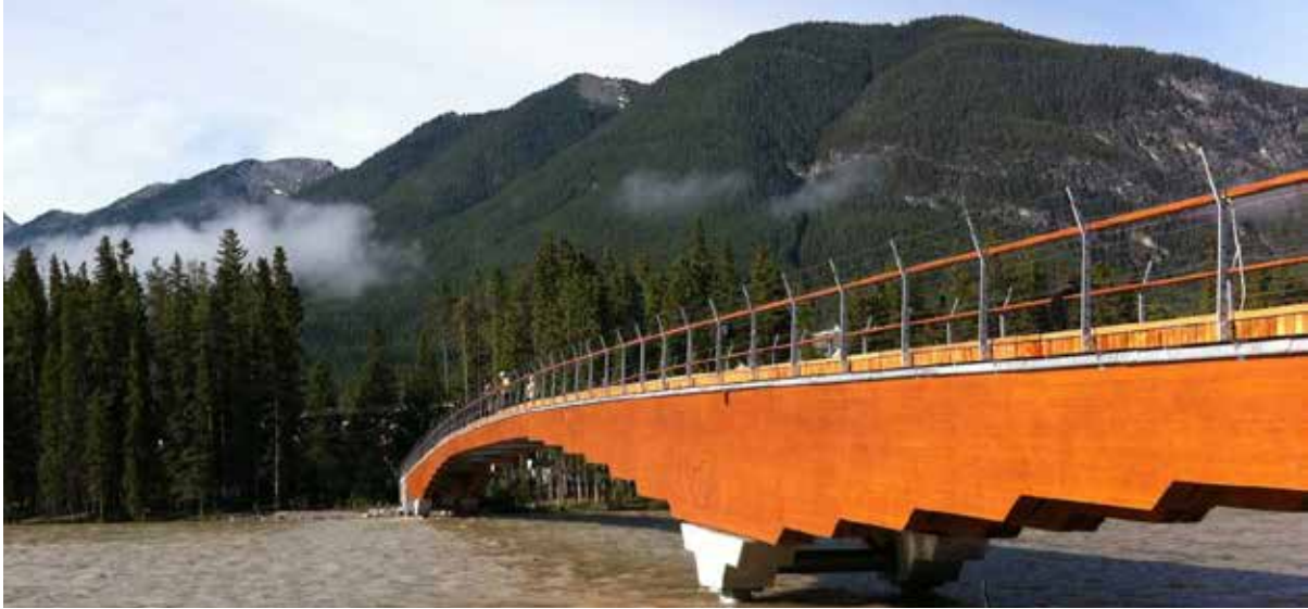
Bow River Pedestrian Bridge and Utility Crossing – 2014 Award of Excellence
