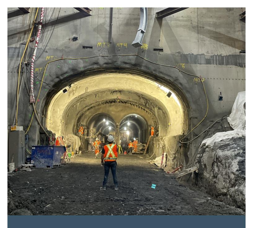
The Mount Royal Tunnel–Double Arch Replacement & Rehabilitation project in Montreal involved a critical 540-meter upgrade of the 5km tunnel for CDPQ Infra. Hatch's design, executed by the CIMA+ HATCH JV (CCH), featured canopy spile replacement for 92 meters and observational repairs for 240 meters. This complex and completely underground work was pivotal in eliminating the double arch concerns from the Réseau Express Métropolitain (REM) transit project's critical path.
